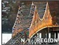
Replacing the Tappan Zee
